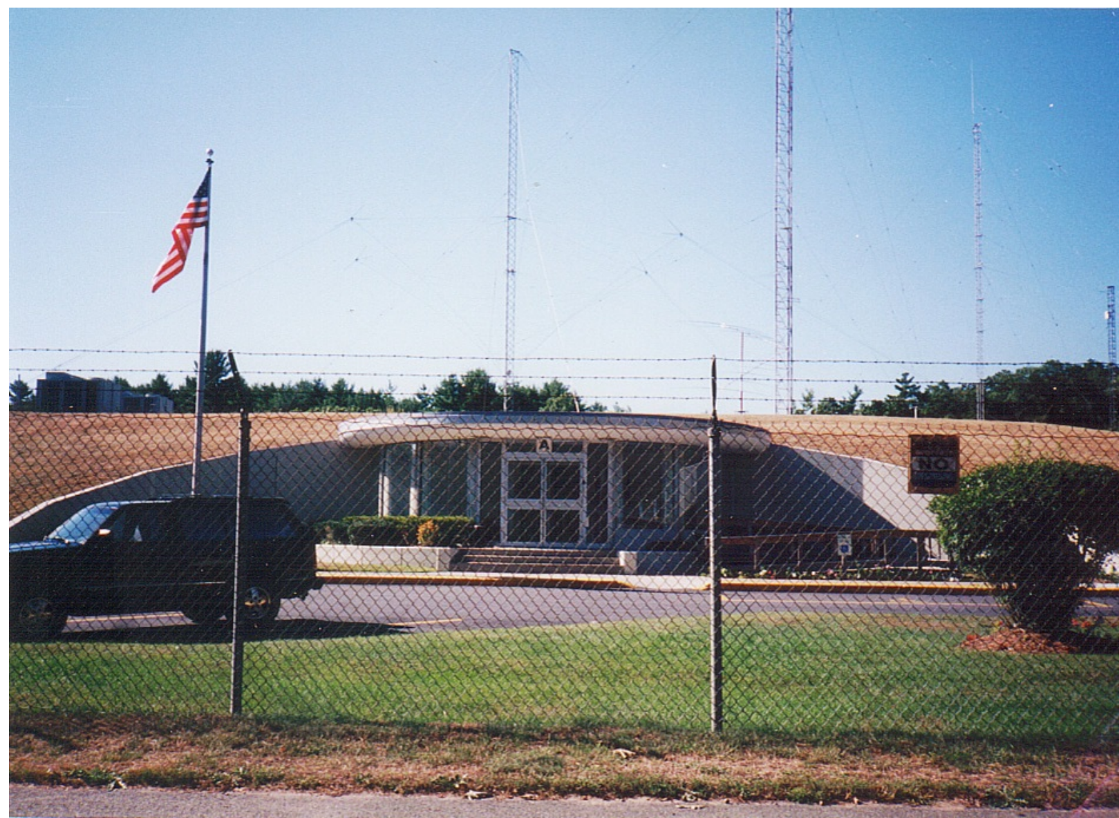
The Federal Regional Center in Maynard, Massachusetts, would have run New England after an attack.
