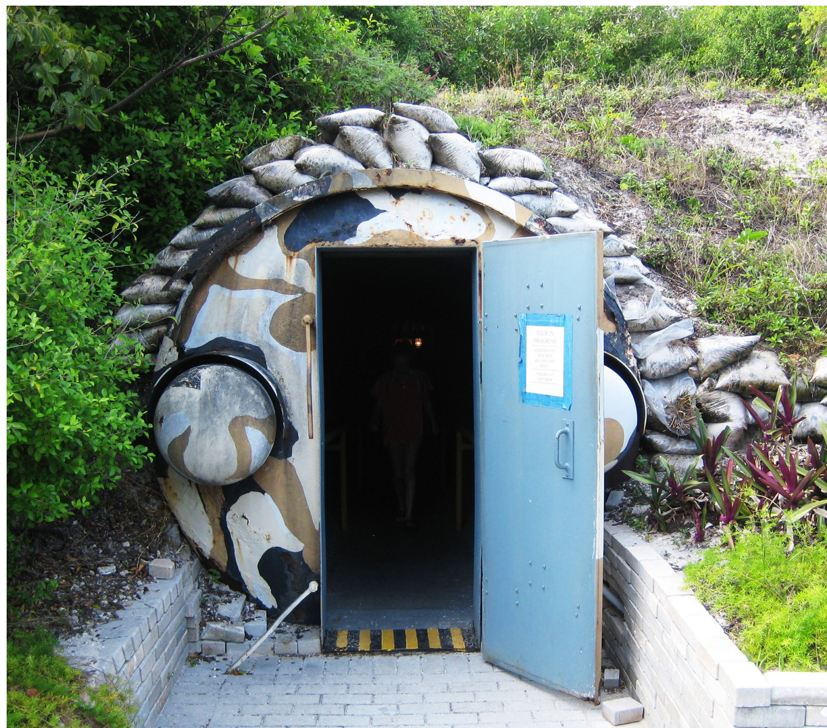
Navy Seabees built this presidential escape bunker on Peanut Island, close to JFK's vacation home in Palm Beach, Florida.
