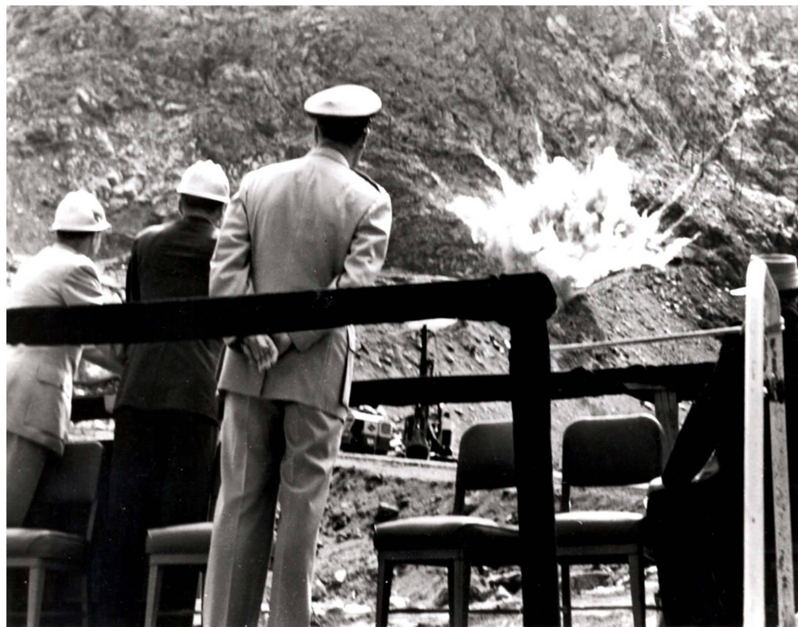
The groundbreaking of the new NORAD bunker under Cheyenne Mountain on June 16, 1961.
