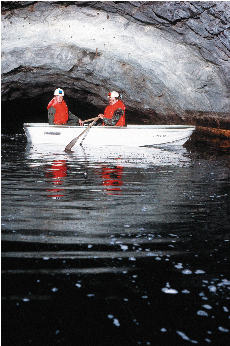
Cheyenne Mountain holds large reservoirs for NORAD's drinking water, heating, and cooling.
