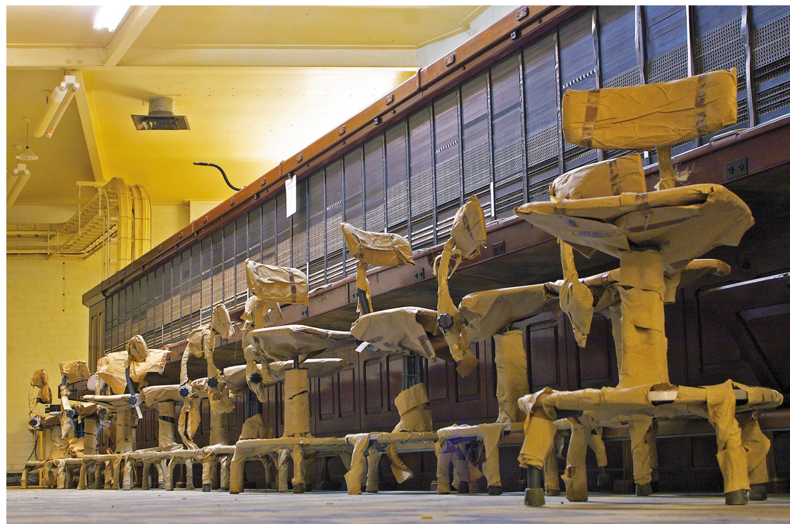
The massive telephone switchboard inside the UK's central bunker, codenamed BURLINGTON, was never used.
