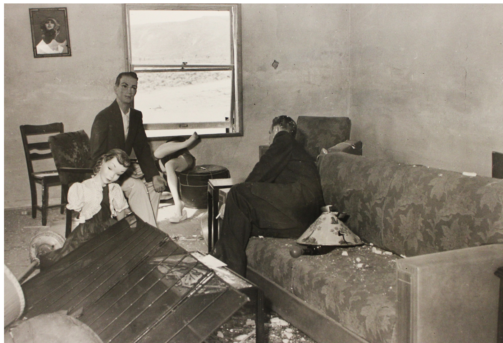
Engineers erected houses and stocked them with mannequins to test buildings' sturdiness to nuclear blasts. The mannequins often fared poorly.
