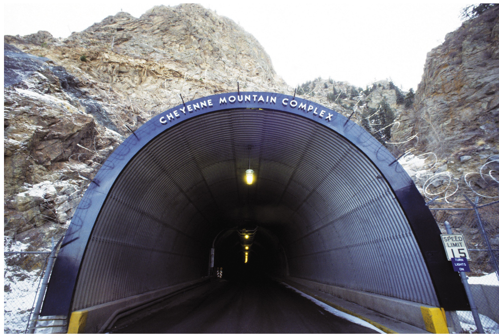
The NORAD bunker served as the heart of the continent's air defenses through the Cold War.
