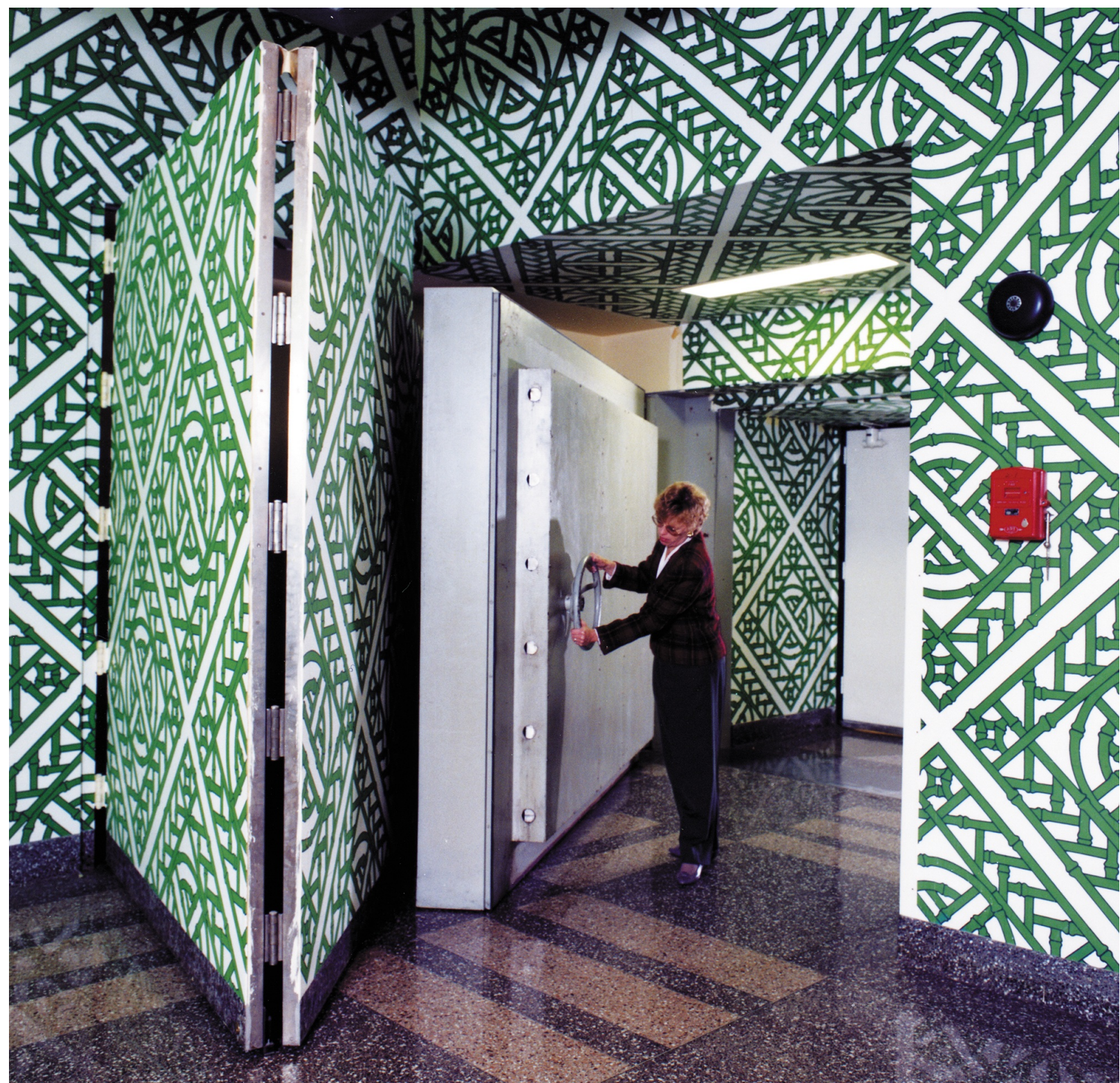
The bunker door was hidden behind a wall in the Greenbrier's conference facility.
